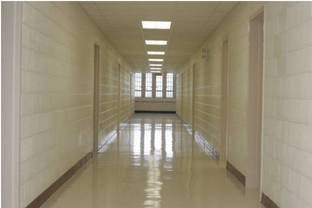
Figure 8. Hallway in Norris Hall
