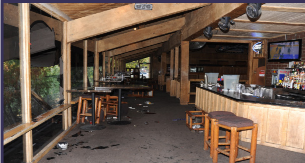
Photo 4: Photo of the glass windows along the north side of the Borderline Bar and Grill.
