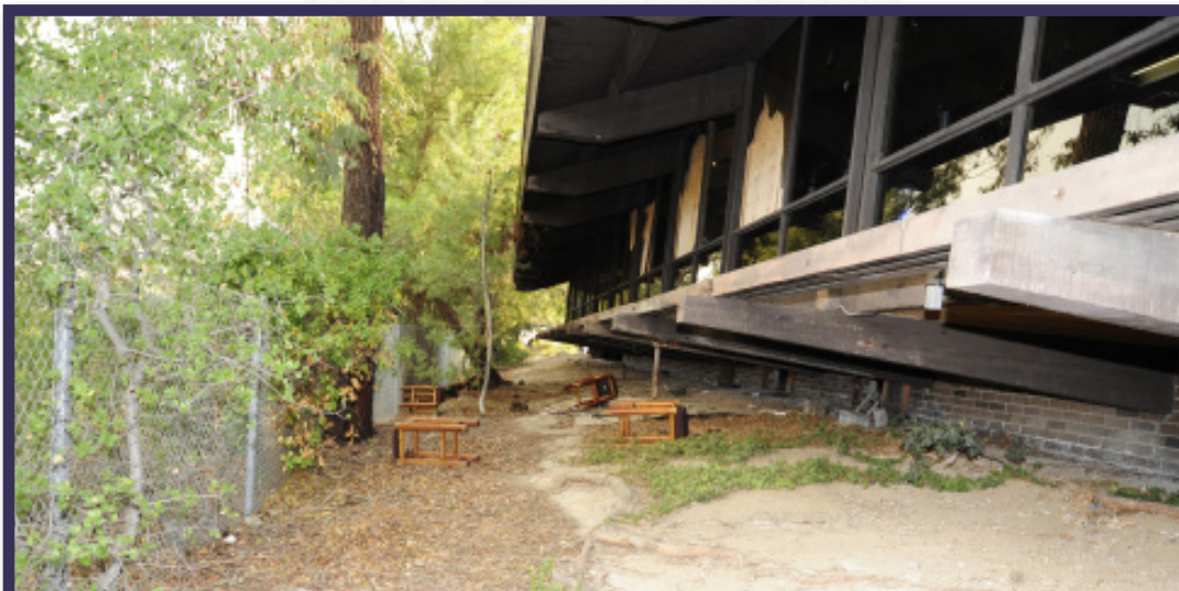
Photo 5: Photo depicts the north side of the bar. This is the location where numerous patrons/employees jumped out the windows. Opposite (or north of) the chain link fence is the on-ramp to the U.S. 101 Freeway (southbound).
